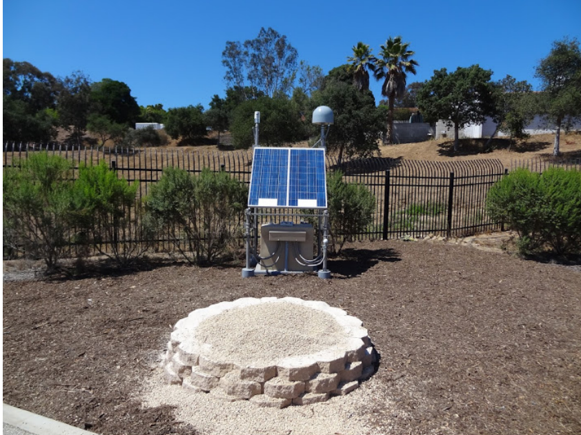
Figure 2. Station EOCG at the Santa Barbara Emergency Operations Center. Seismic vault is located in the foreground. Photo courtesy of Dan Determan, USGS. Photo was taken sometime between July and December 2014.
